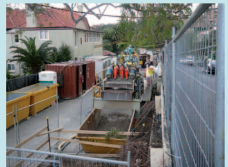
The tight and compact drill site.
